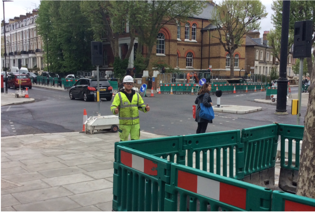
Local safety scheme, junction of Sutherland Ave and Shirland Rd.
